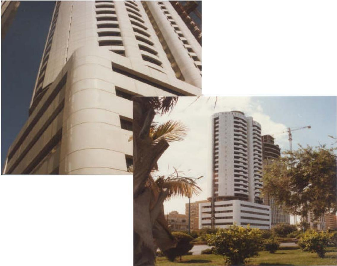
Figure 6: Corniche Towers, Abu Dhabi: nearly 10,000 m<sup>2</sup> of GRC has given 20 years of trouble-free performance in the Middle East's hot, salty and sandy environment.
