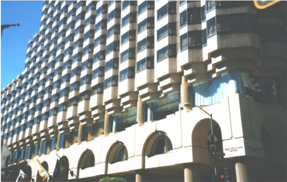
Figure 4: Parc Fifty Five, San Francisco. A variety of sculptured panels were created in GRC – from fluted, circular and oval column covers to delicately combed, three-dimensional spandrel panels and large arches with deep rustic joints: 3624 GRC panels cover 17,000 m<sup>2</sup> in total.
