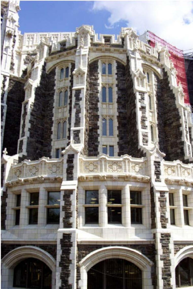
Figure 5: The reconstruction of the exterior of Shepard Hall, built in 1907, is a multi-phase project that will eventually lead to the replacement of 72,000 units and over 4000 shapes, including many ornate sculptures. The project is still on-going and it is a tribute to GRC that many of the new elements are being fixed next to 10-year-old pieces with no discernable differences being visible.
